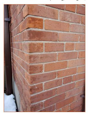
Image 24. View south showing the common bond brick pattern of the main house
