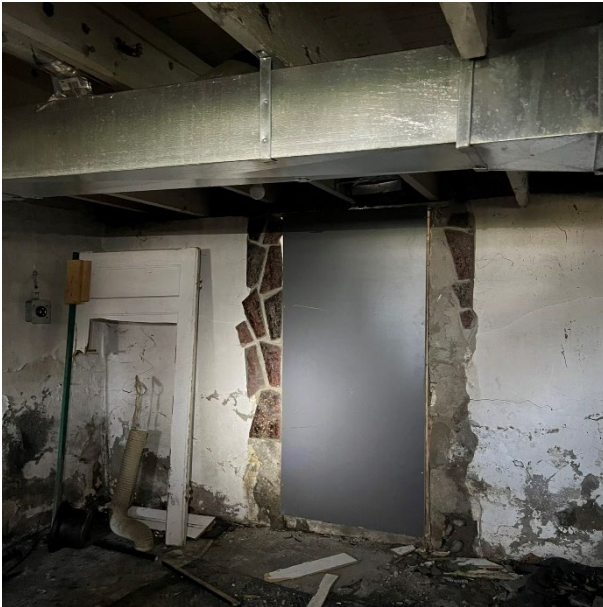
Closed Basement Entrance to Yard
