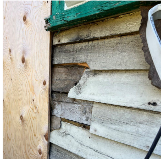
Exposed Original Wood Siding
