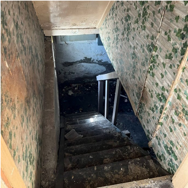
Stairwell to Basement
