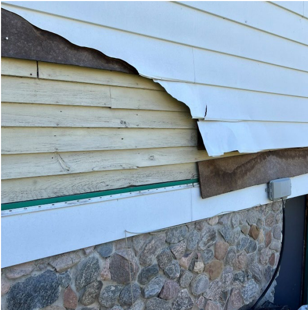
Exposed Original Wood Siding
