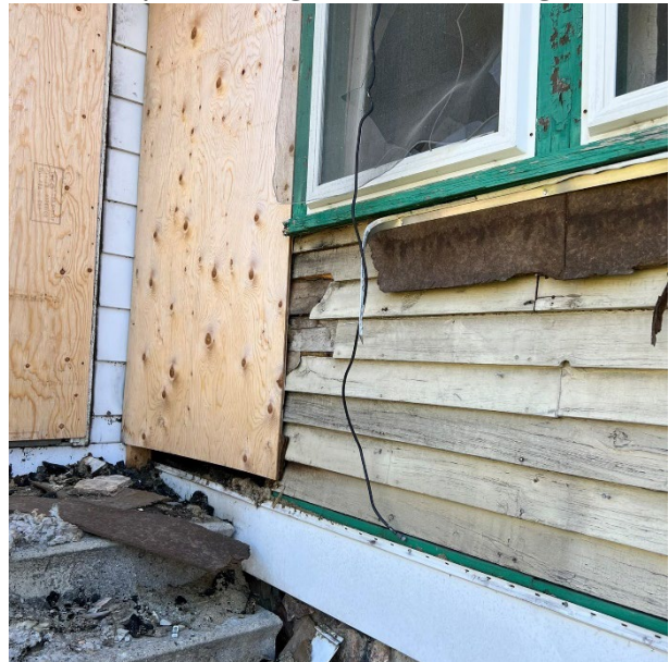
Exposed Original Wood Siding
