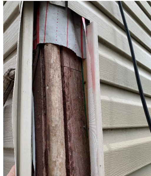
Fig.12: The original wood cladding (MHBC, 2022)
