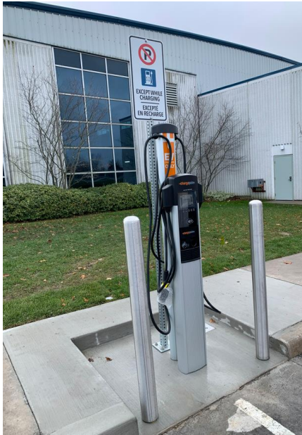
Figure 10 Level 2 EV Charging Station at McKinney Centre
