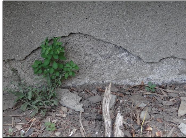
Figure 17: Spalled concrete foundation
