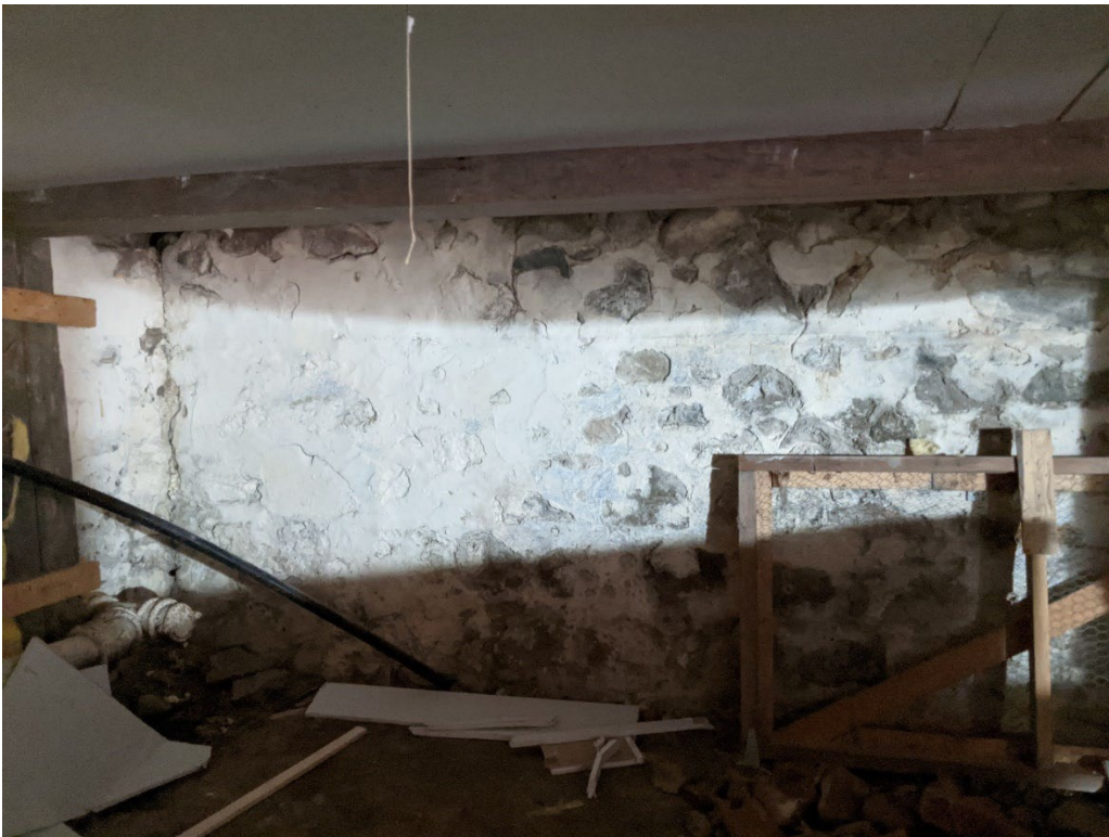
Figure 28: Fieldstone and mortar wall, located in basement (CY 2020).
