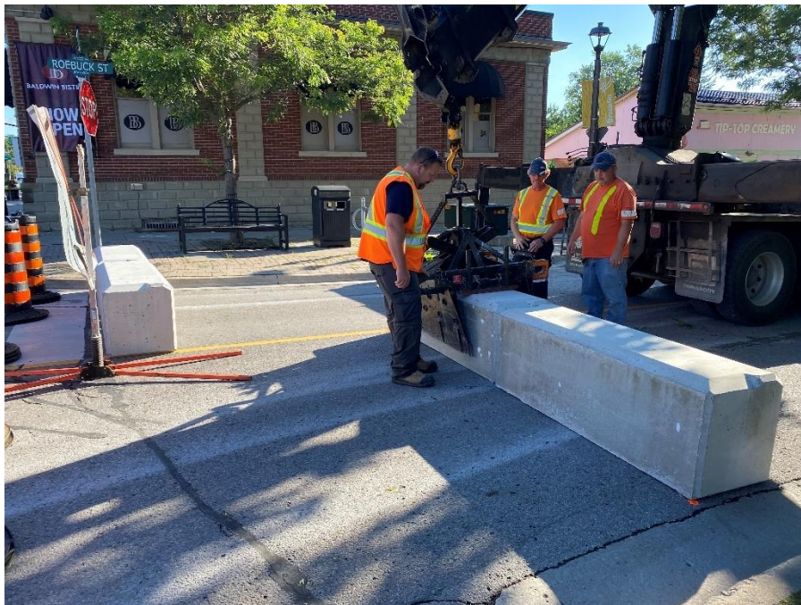
Figure 2 – Installation of concrete barriers for road closure
